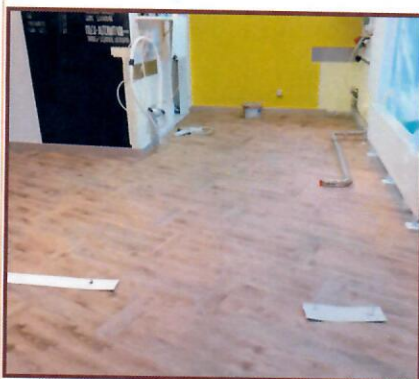
The new Café renovations include a brand new floor!
